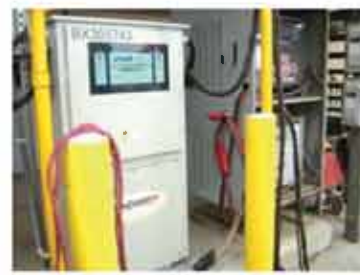
FED FROM (E) DIST. BD. BC7S, CIRCUIT 2
