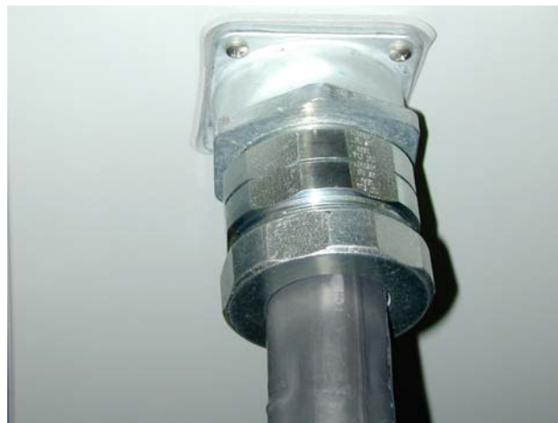
Figure 4.6 Installed Cable
