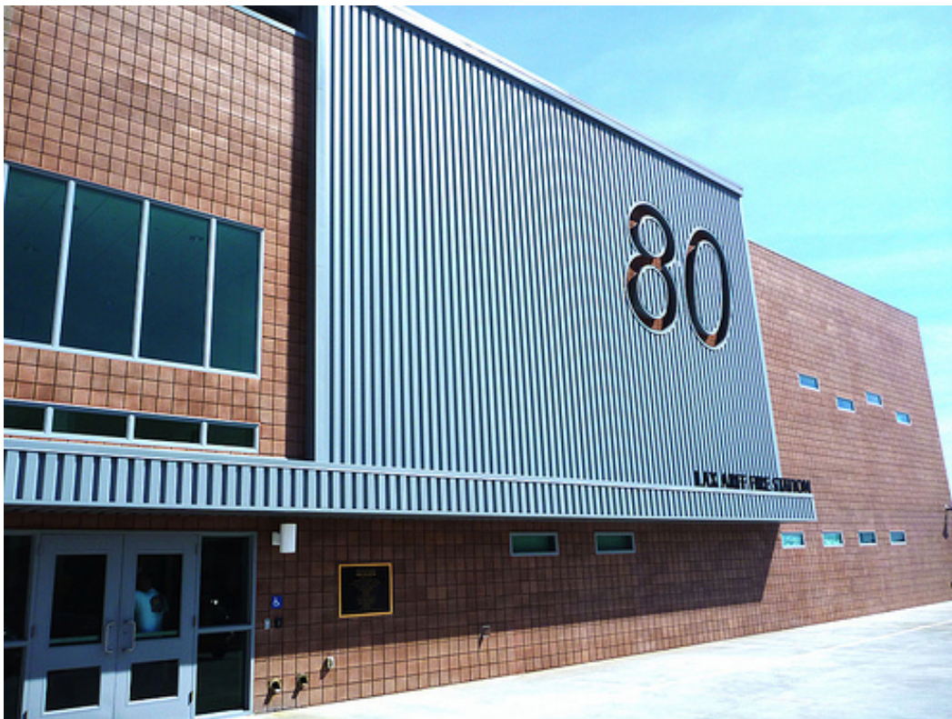
Figure 1.2.2-1: Aircraft Rescue & Firefighting Facility (Photo courtesy of Clay Irving)
