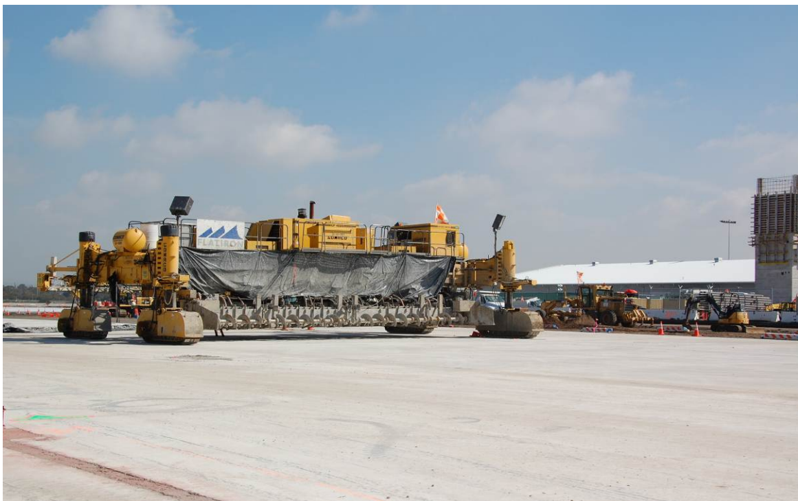
Figure 1.2.3-1: Taxiway S Under Construction at LAX
