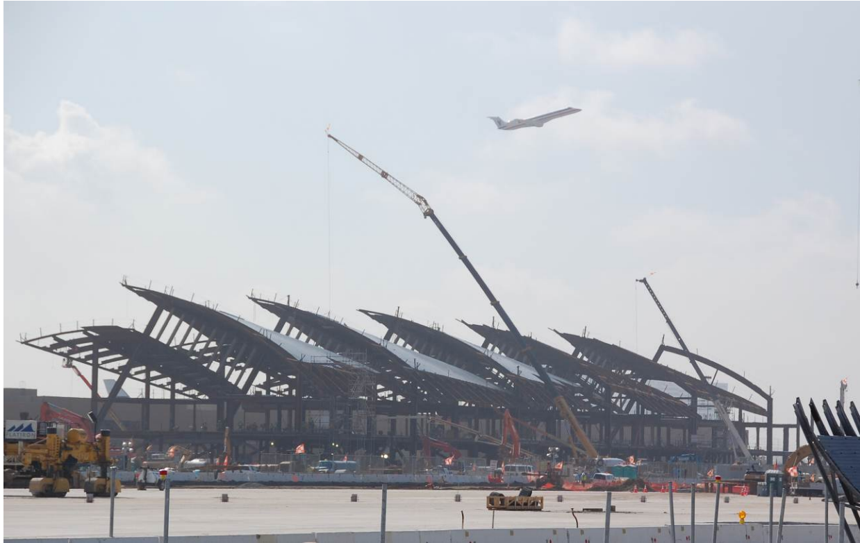
Figure 1.2.4-1: Bradley West Project Under Construction at LAX
