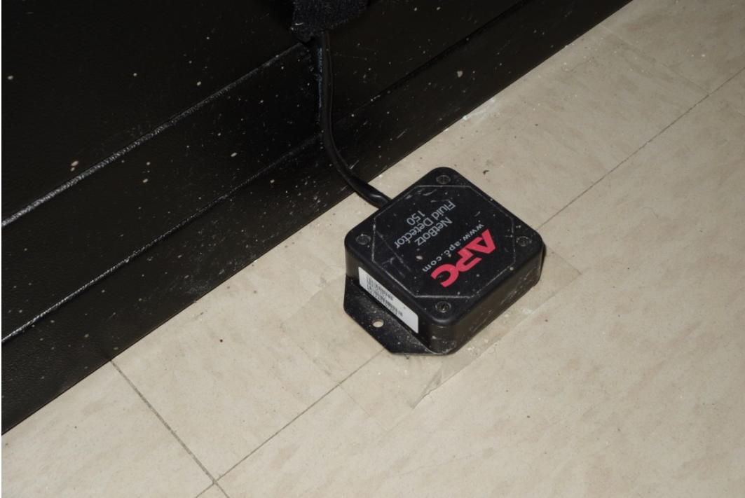
Sample Netbotz floor-mounted flooding sensor.
