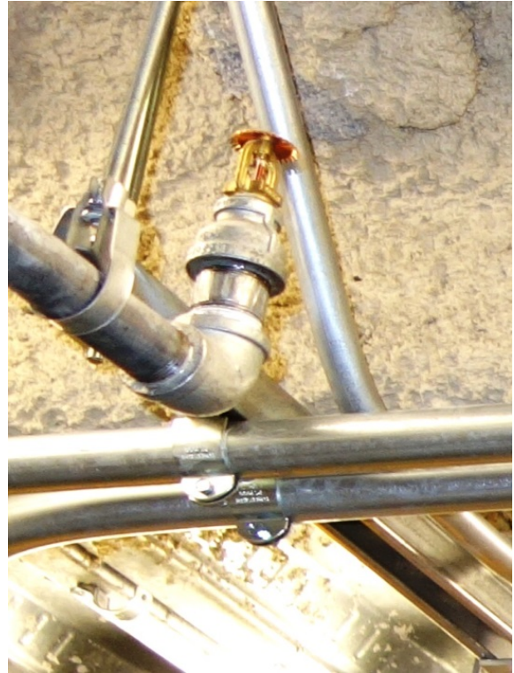
Sample IT Room sprinkler heads.
