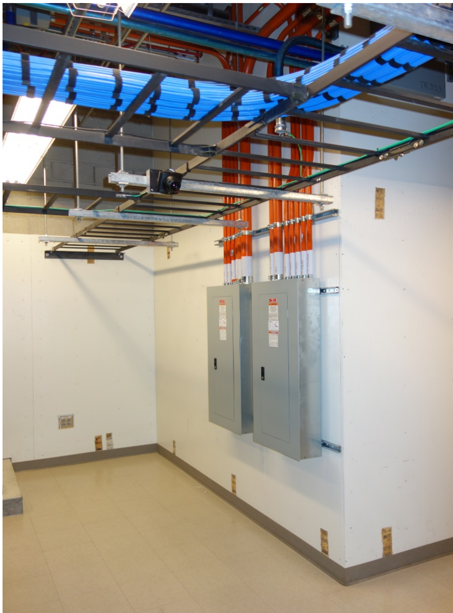
Fire-rated plywood stamps shown unpainted on painted plywood backboard.
