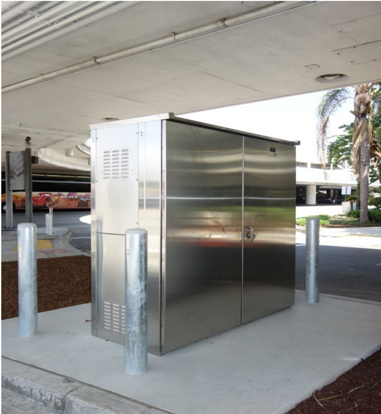
An outdoor TE with top and bottom vents on both enclosure sides.
