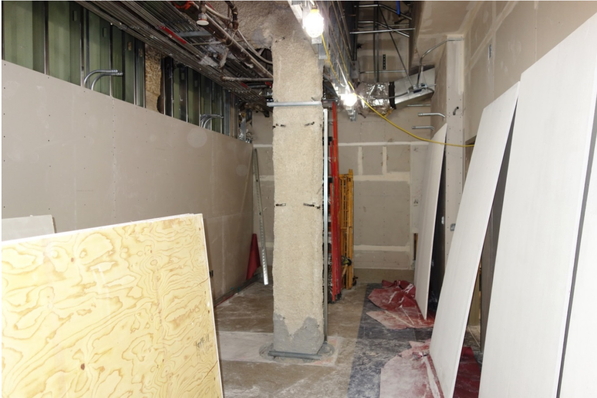
A standard rectangular IT Room Layout upsized due to unavoidable column interference.
