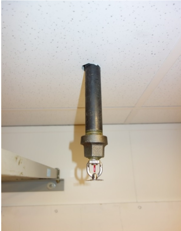
Sample IT Room sprinkler heads.
