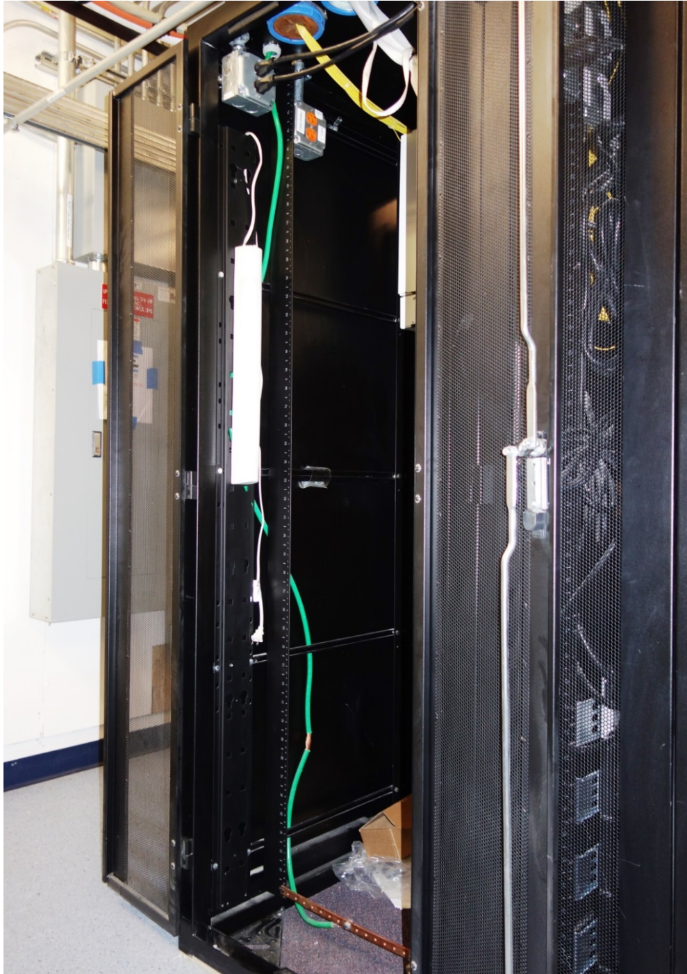
Cabinet light fixture can mount on the side to avoid top obstructions.
