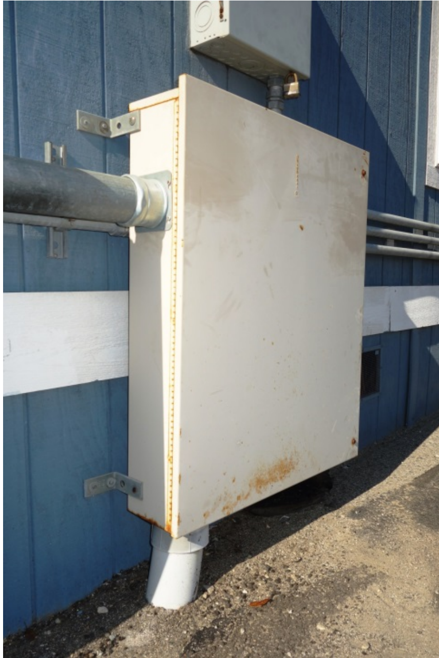
Legacy TE showing two 4-inch conduits on the left plus additional conduits on the right.
