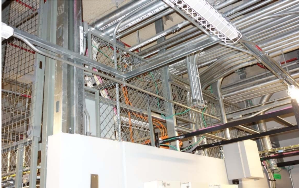
New construction showing a 14'+ open ceiling for easy access to conduit.
