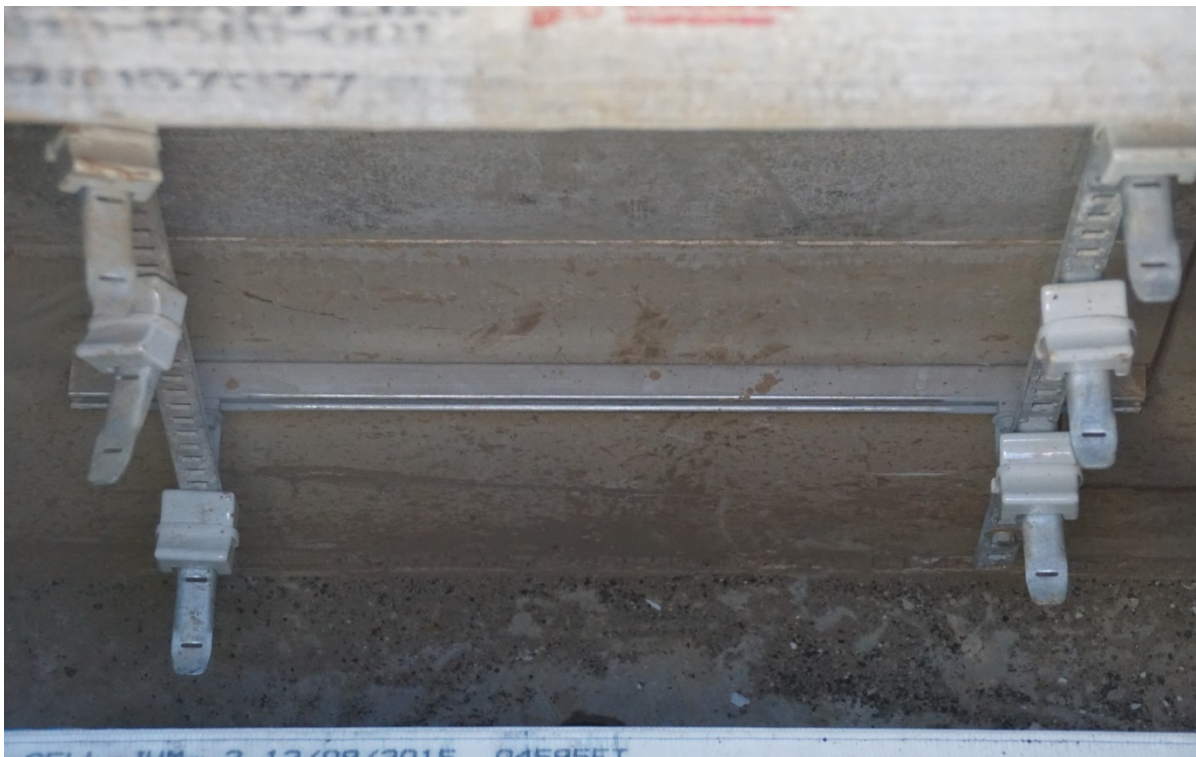
Maintenance Holes require cable mounting racks on both sides able to support 400 lbs each.
