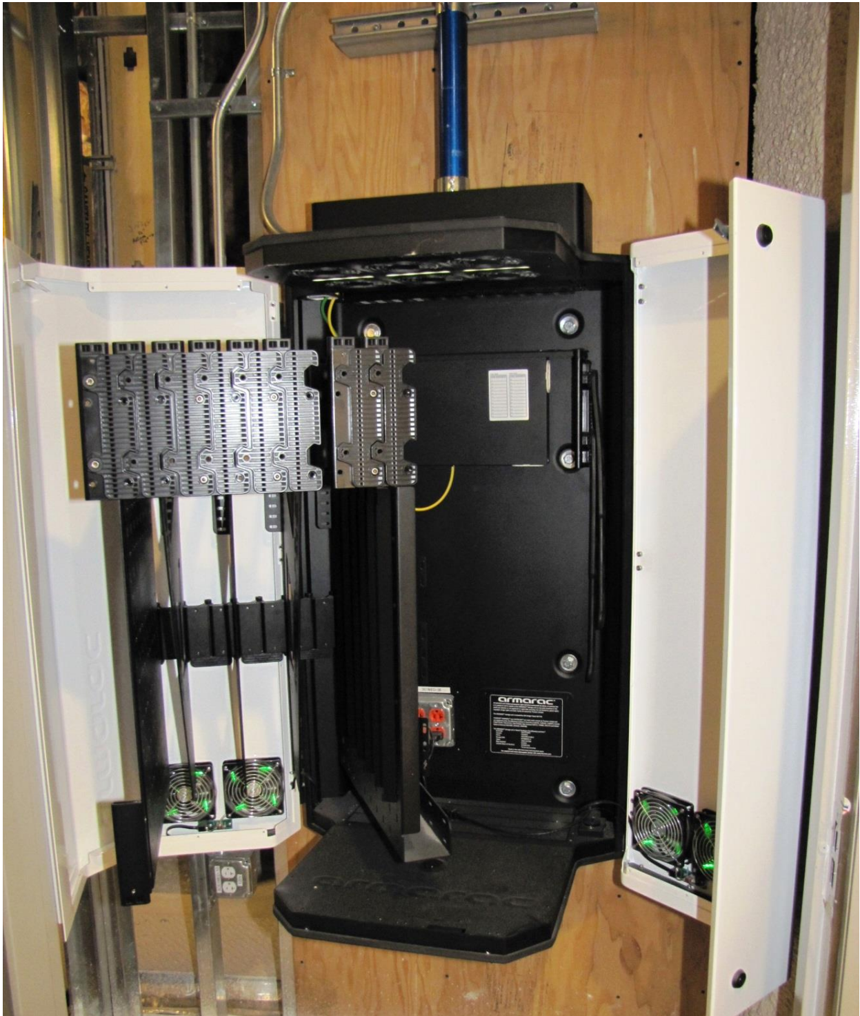
Armarac TE inside view showing swing-out panels for vertically-mounted equipment.
