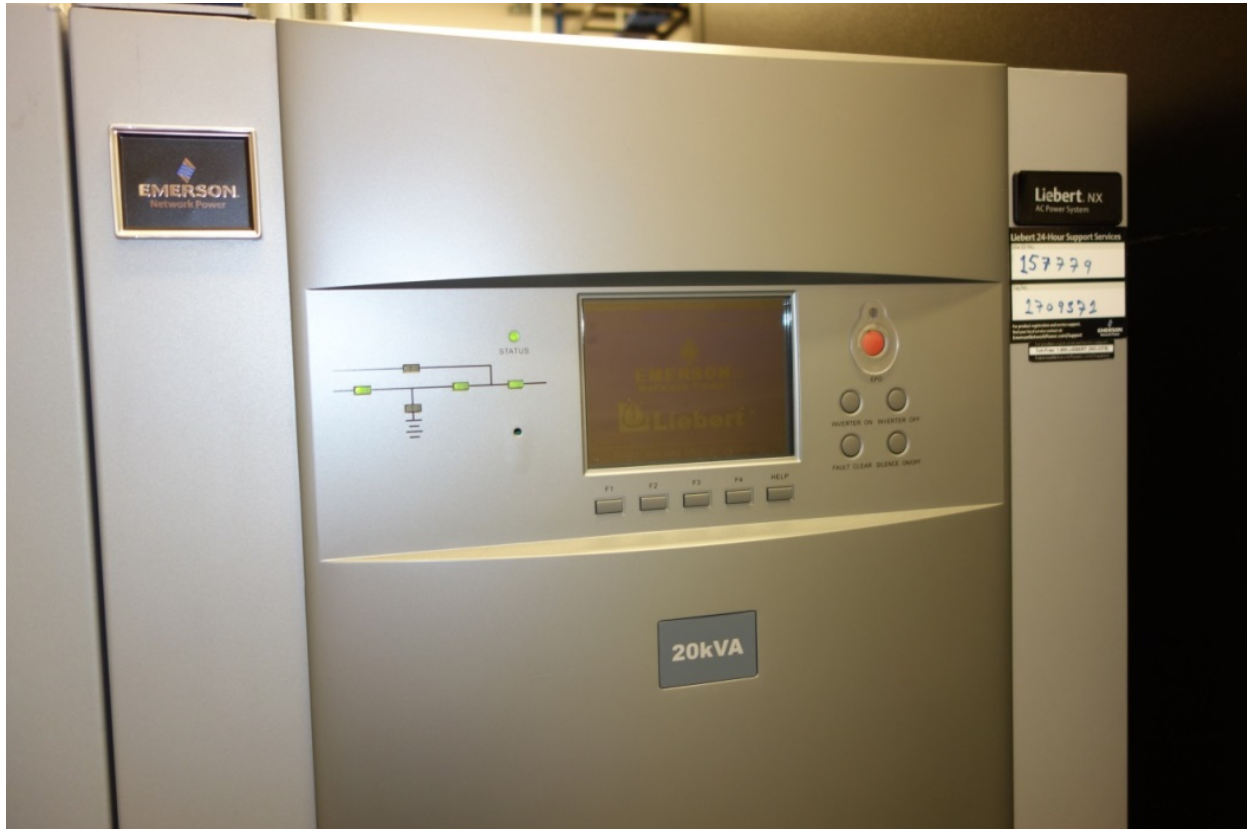
Close-up of a 20kVA Liebert UPS for a standard 6-cabinet IT Room.
