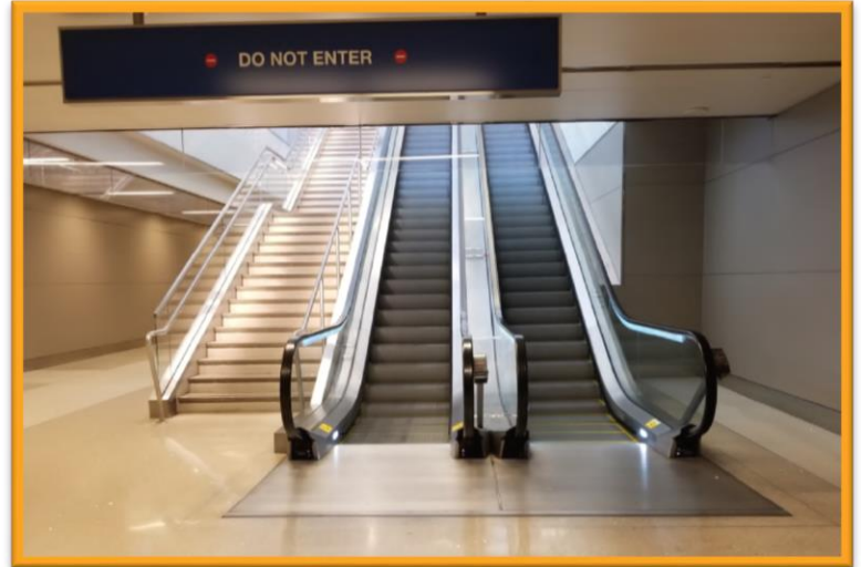
Gate 148 Escalator Terminal B
