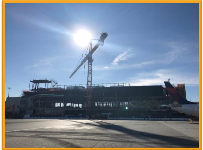
Terminal 1.5 from airside
