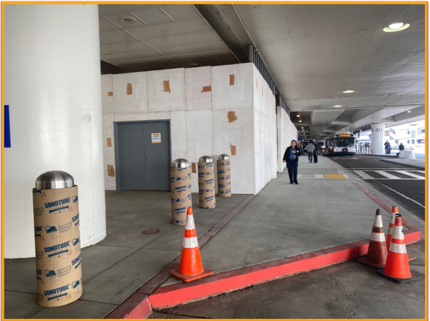
Terminal 4 / 5: Temporary Sidewalk
