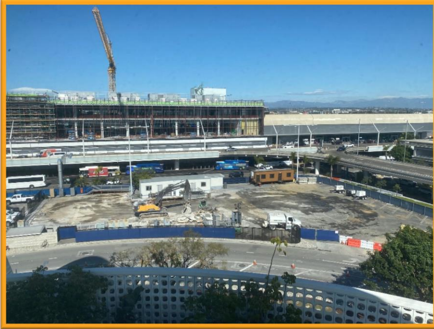
Surface Lot 2 Trailer Demolition with Terminal 1.5 in background
