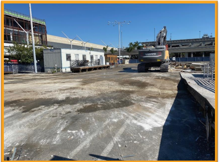
Surface Lot 2 Trailer Demolition
