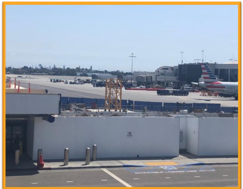
As of Monday, April 20, 2020, only the base was constructed
