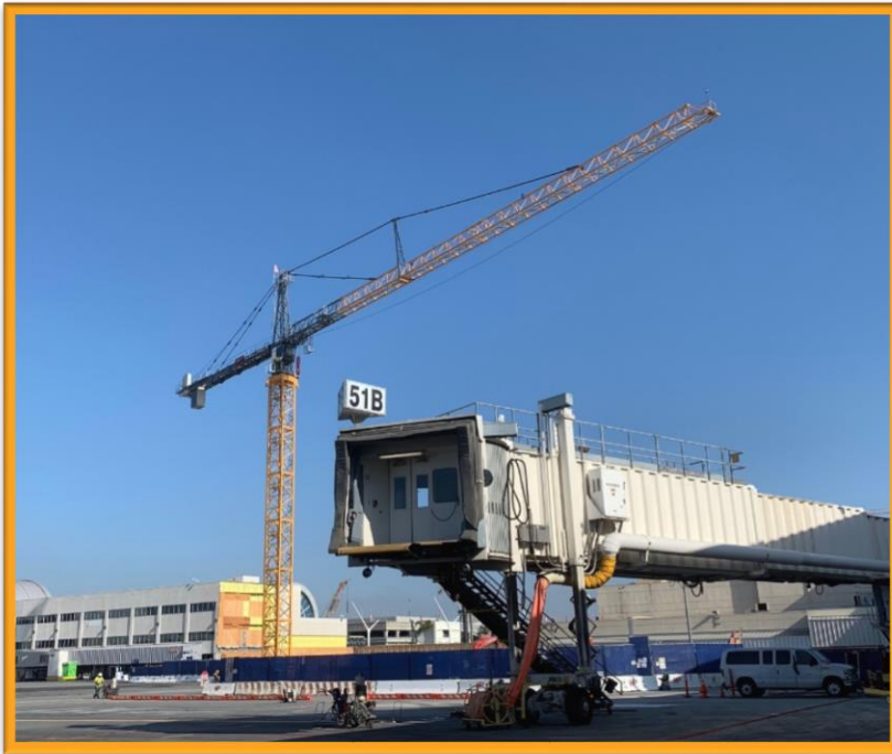
Terminal 4.5 Tower Crane full built as of Monday, April 27, 2020
