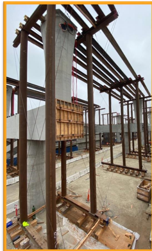
Both photos showcase the guideway falsework currently being constructed at the future East CTA Station site for the Automated People Mover
