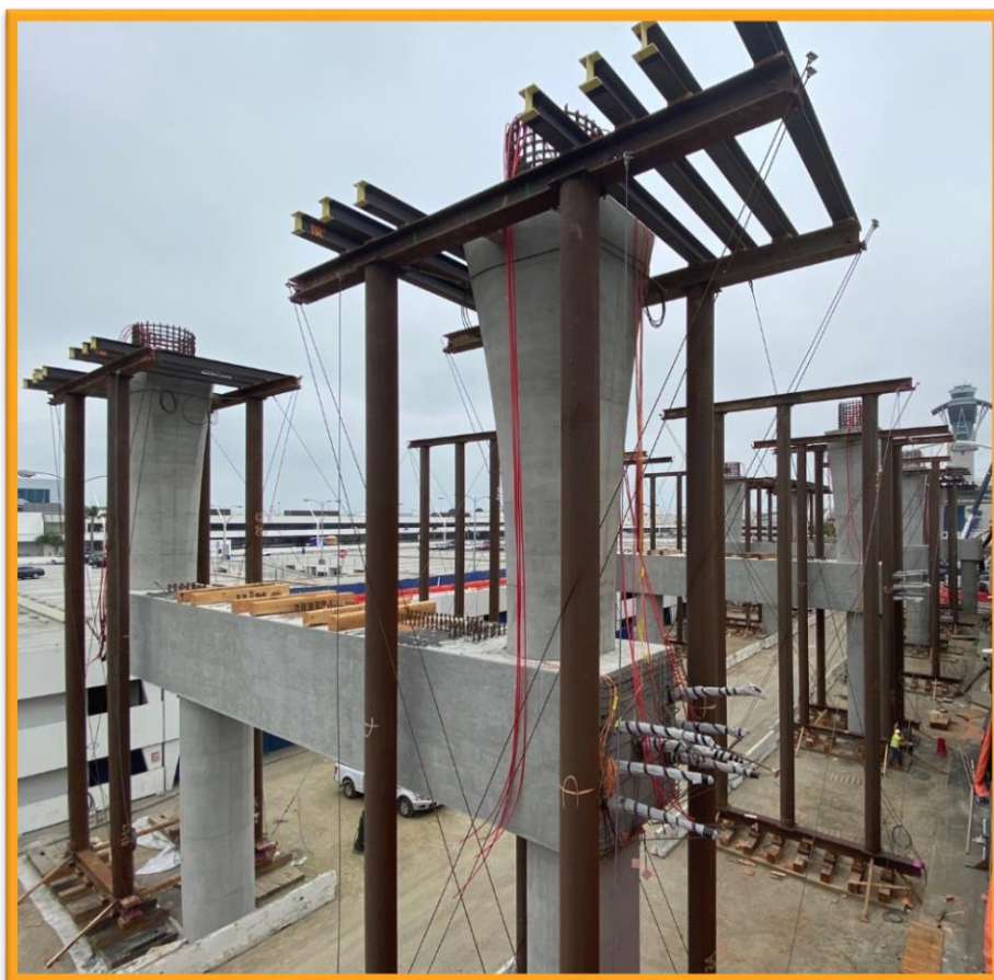
Both photos showcase the guideway falsework currently being constructed at the future East CTA Station site for the Automated People Mover
