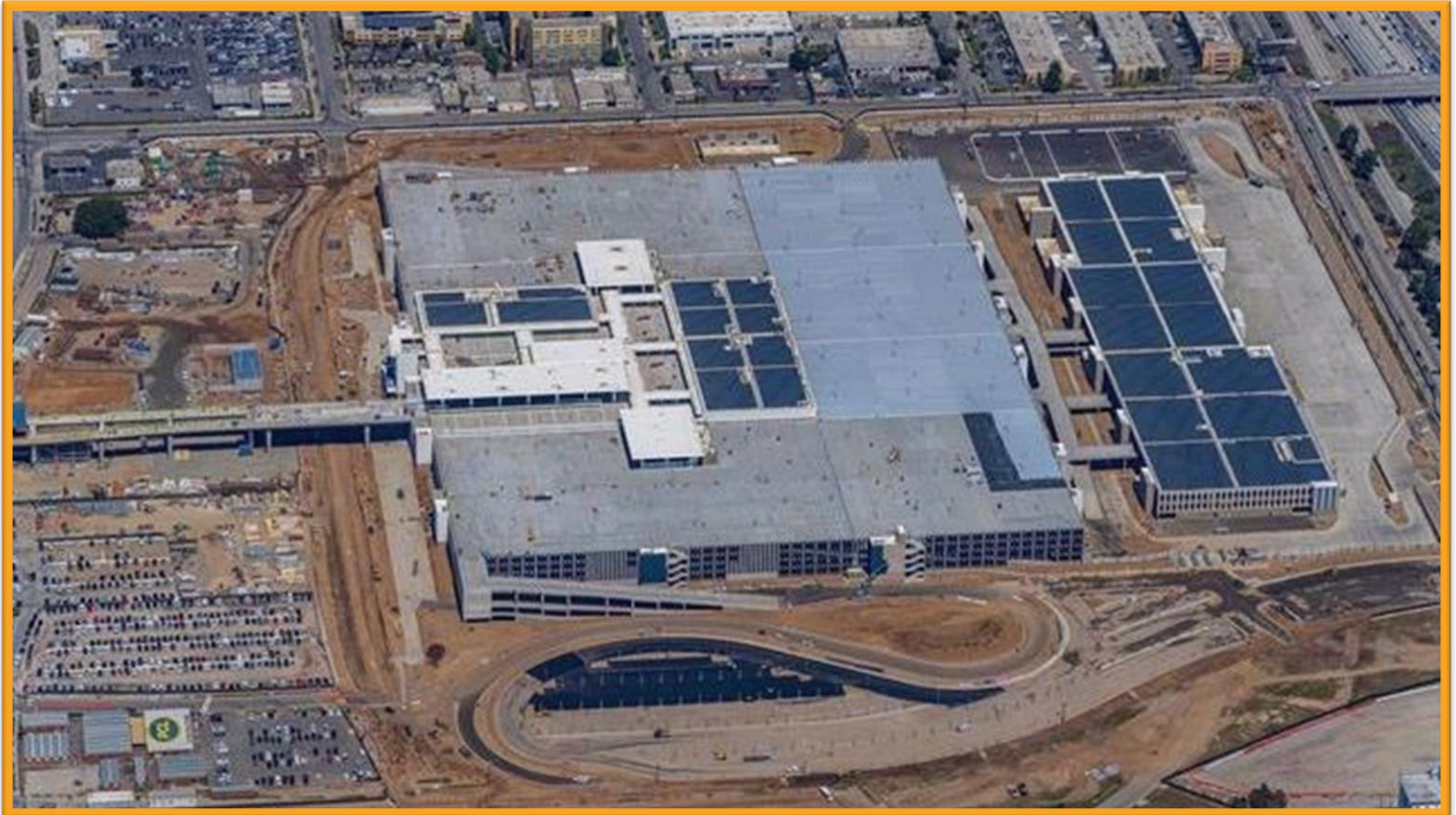
An aerial view of the LAX ConRAC Facility with Arbor Vitae St to the north, Century Blvd to the east, and the Automated People Mover guideway at the facility's west side
