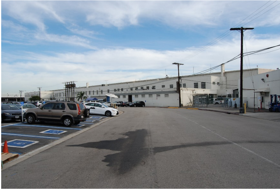
Intermediate Terminal Facility (#133, 6000 Avion Drive, 1945-1947)
