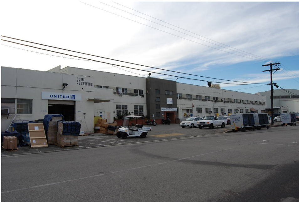
Intermediate Terminal Facility (#134, 6010-6024 Avion Drive, 1945-1947)
