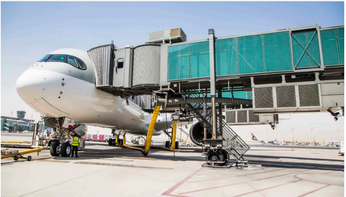
Qatar Airways Airbus A350 connected to pre-conditioned air supply at Hamad International Airport
