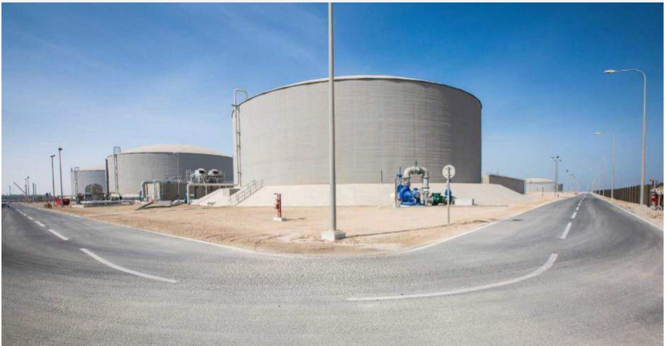
Hamad International Airport waste water treatment plant
