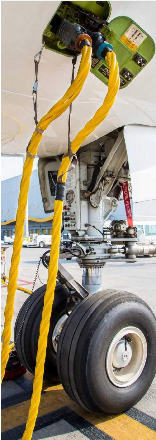
Fixed electrical ground power
