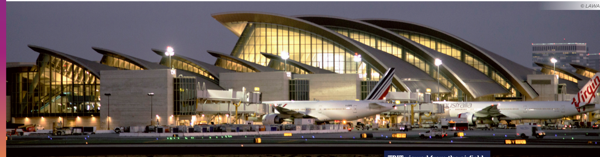
TBIT viewed from the airfield
