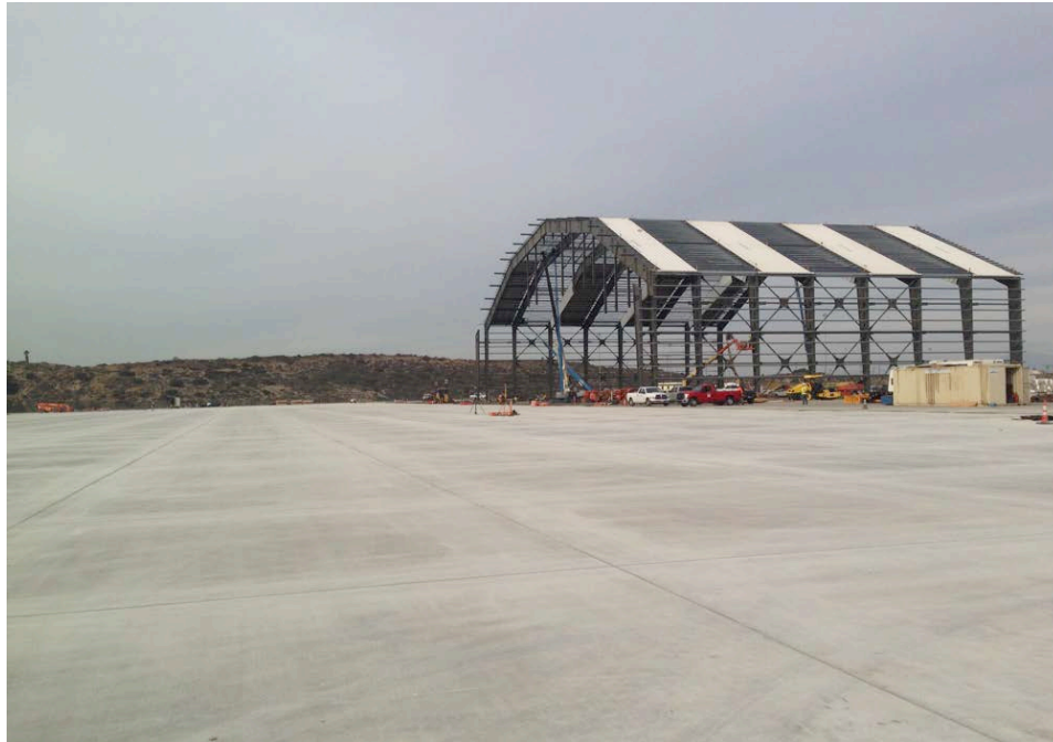
Figure 1.2.3-1: Qantas Hangar Construction Site
