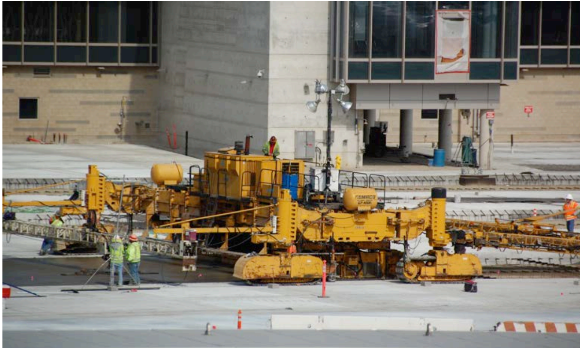
Figure 1.2.1-2: TBIT – East Apron Construction Progress – Heavy-Duty Paving Equipment in Use
