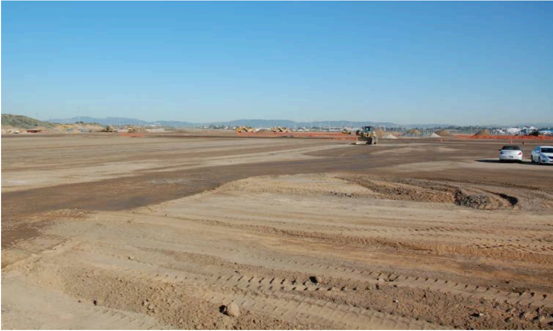
Figure 1.2.2-2: WAMA Construction Site
