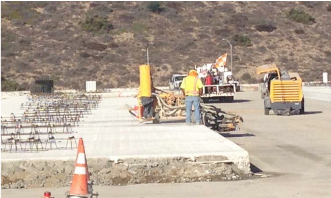
Figure 1.2.2-3: WAMA Construction Progress
