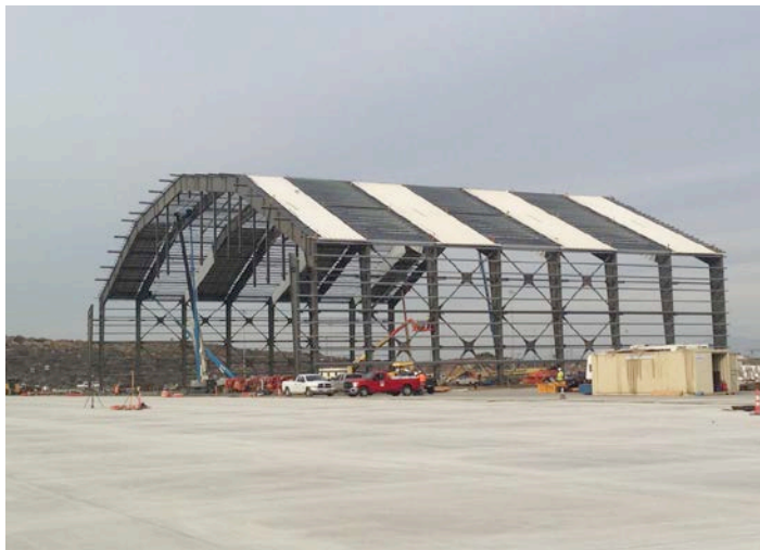
Qantas Hangar Construction Adjacent to WAMA Site
