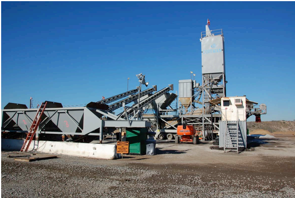
Figure 3.3-1: Batch Plant Operations on WAMA
