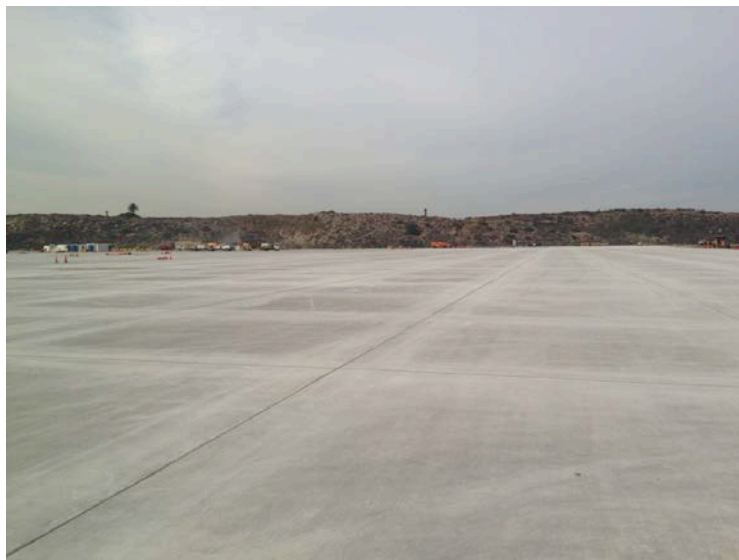
Paving Substantially Complete at WAMA Construction Site as of December 2015
