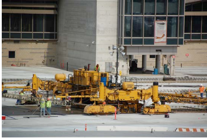
Paving Equipment Operating at TBIT Renovation – East Apron
