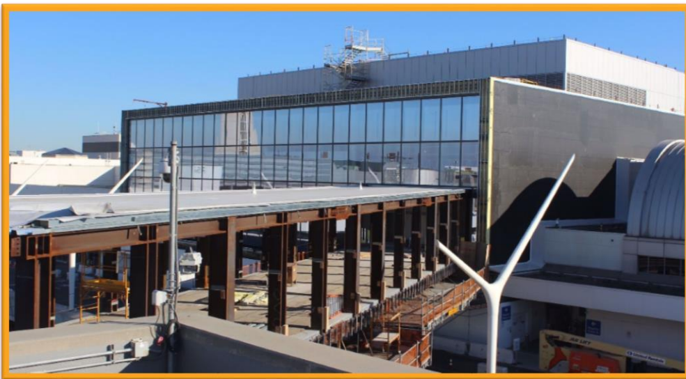
Current progress on Terminal 4.5 February 2022
