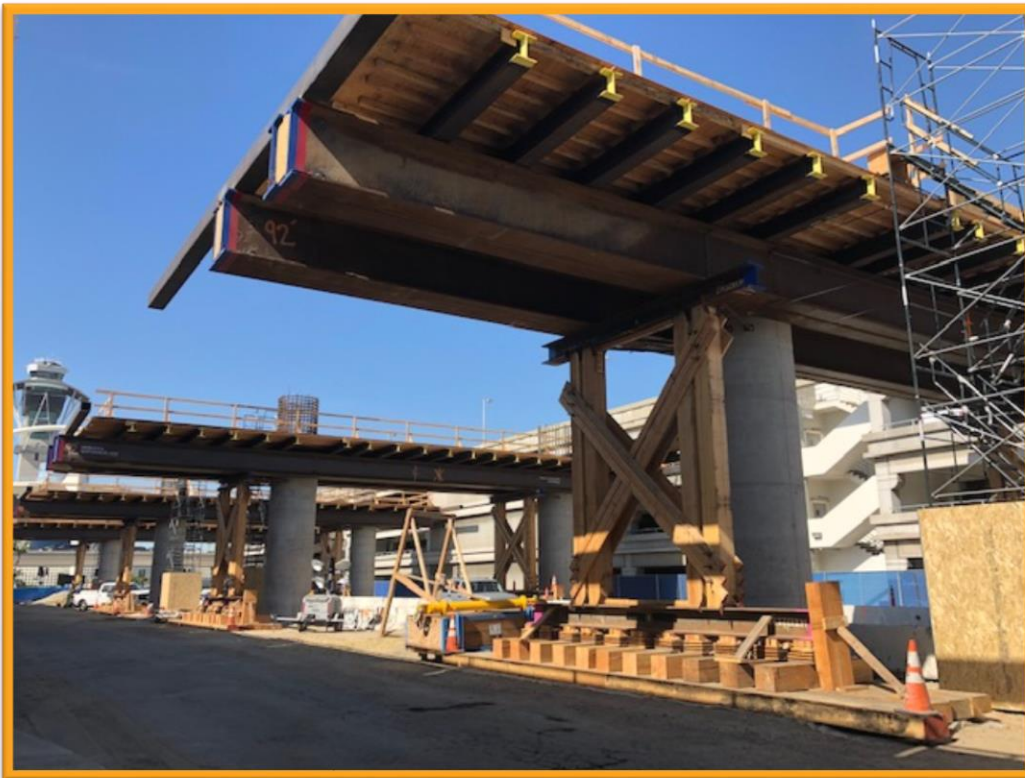
Foundation piles and falsework on Center Way for the APM Project
