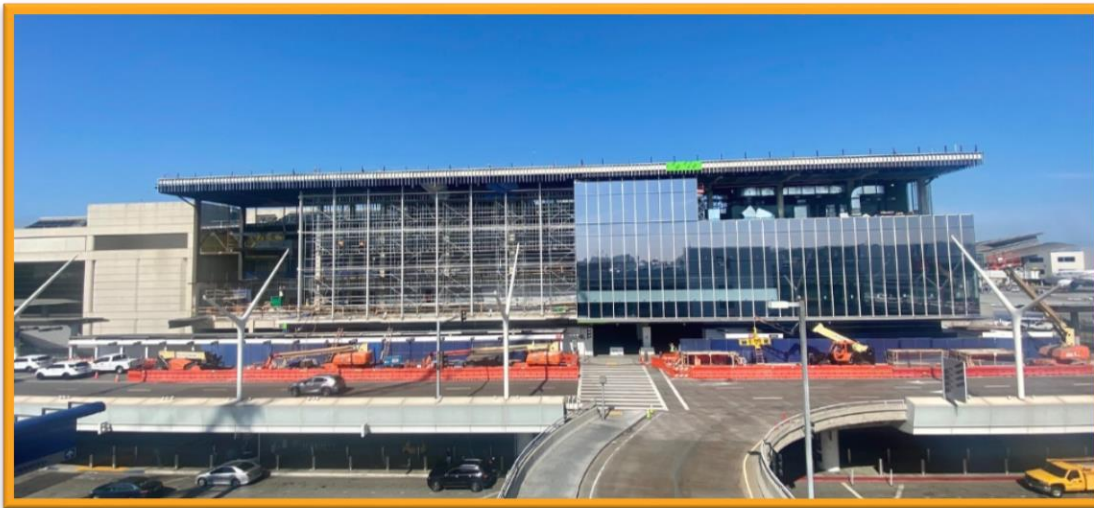
Glass installation progress at Terminal B's north end
