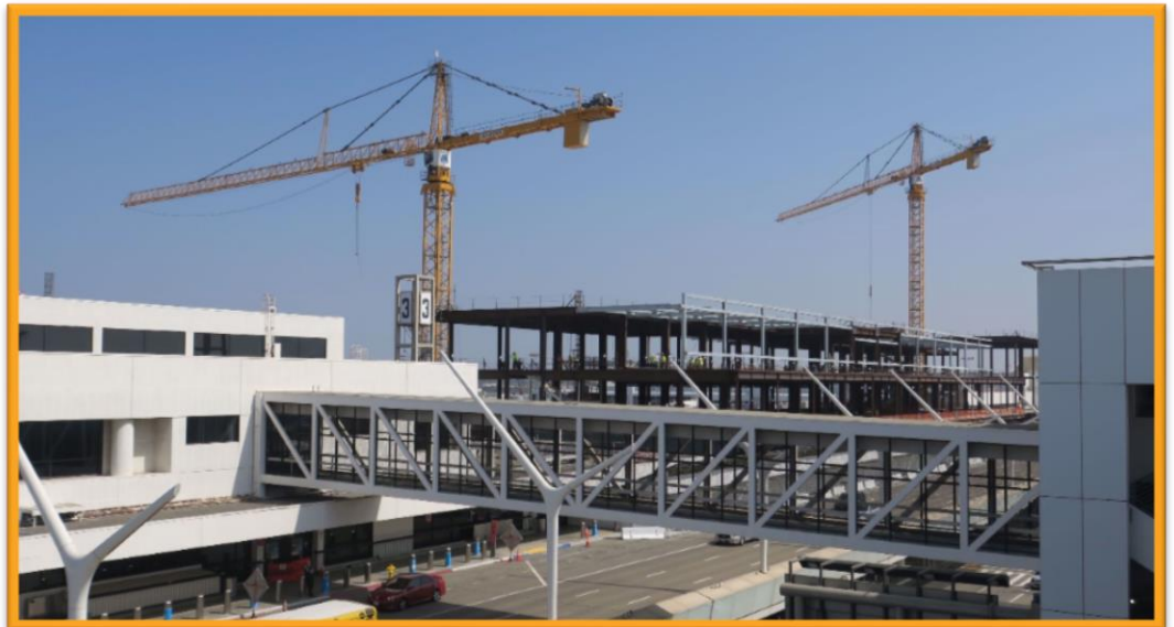
Terminal 2 / 3 Head House Construction & Terminal 3 Ped Bridge to be Demolished
