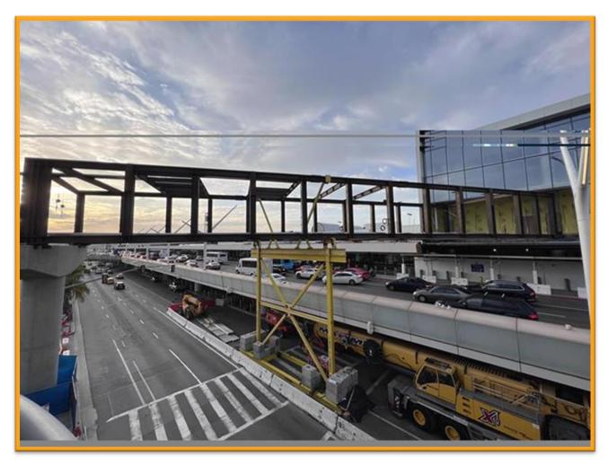
"Terminal 5.5" Pedestrian Bridge with yellow shoring tower supporting construction. The shoring tower will be removed this week and the Arrivals roadway lanes (pictured closed) will be re-opened
